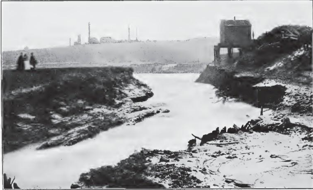
Marshall's brine shaft; Worthington's & Cheshire Amalgamated; Ashton's pumping water station. The cascade is from an old hole behind the sinking that was taking place, when Ashton's works fell and the water dropped. The water is seen running away from top of brook the wrong way. Photo taken looking across Dunkirk, Northwich.
